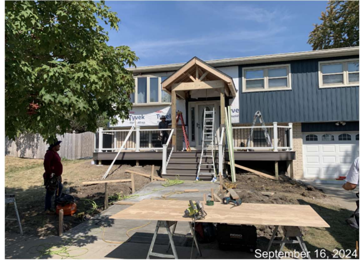
During construction (September 2024)
